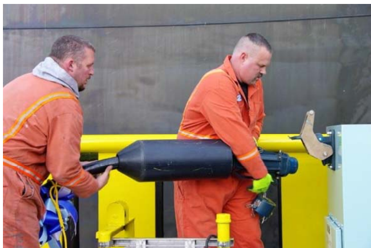
Workers connecting a vessel at the TOTE Terminal to shore power.
